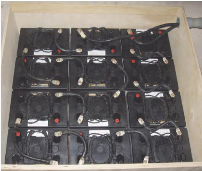
Figure 80: A BESS array of 12 batteries
