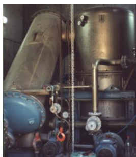
View of the geothermal unit desalination plant of Kimolos. The condenser on the left and one evaporator on the right side
