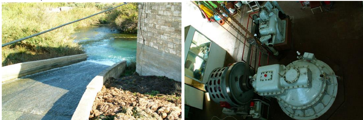
Figure 50: A micro hydropower plant in the island of Crete (MYHS Almyros, Chania Crete, Greece) 63
