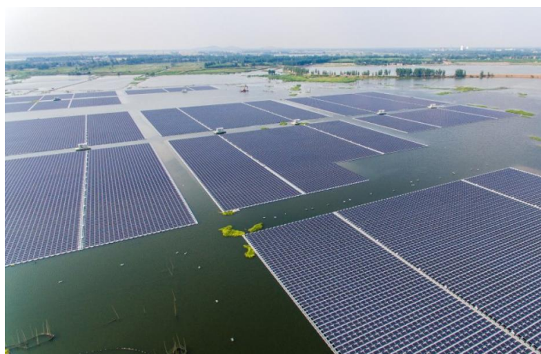
Figure 29: The floating solar farm in Huainan, China is made up of 160,000 panels, attached to each other in a huge mosaic structure 27 . ©STR / AFP
