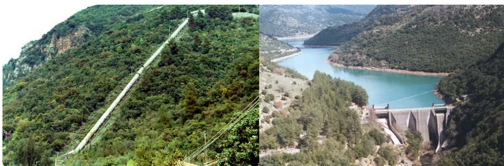
Figure 49: A typical medium size Hydropower plant with reservoir. Penstock (left) and Dam (right) (MYHS Ladonas, Greece) 62 .
