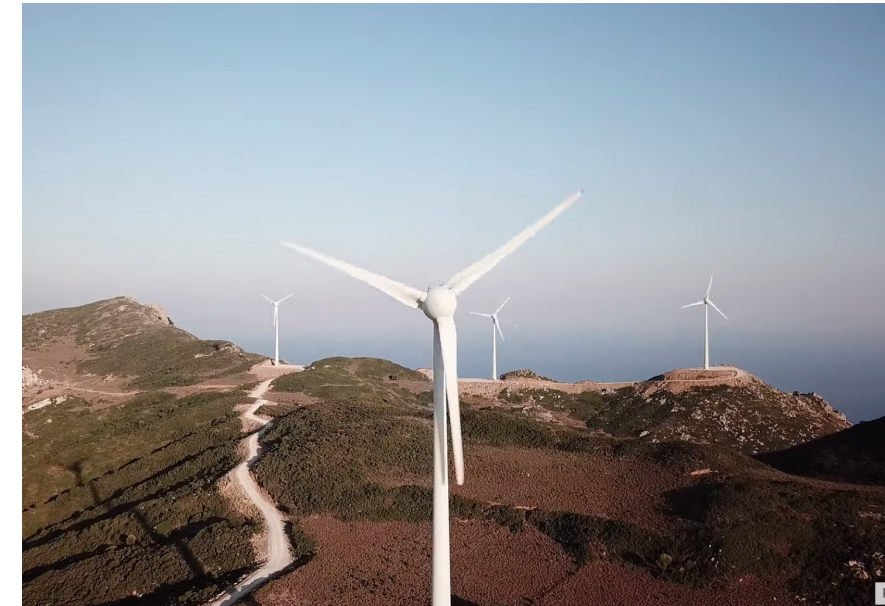
Wind turbines on Kos island (Source: sani)
