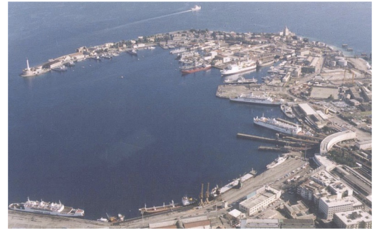
Aerial view of the Port of Messina
