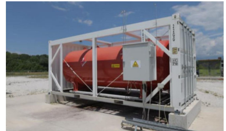
12 m 3 hydrogen tank used in the REMOTE demo site Agkistro, Greece (Source: Documents sent to NESOI)
